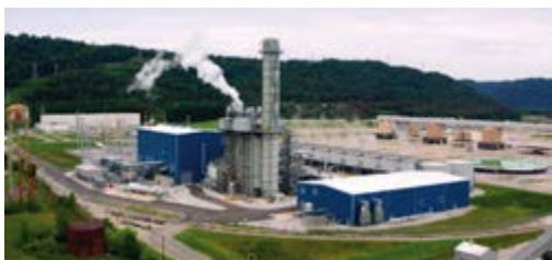
Figure 3: Long Ridge Energy recently converted its 485-MW, natural gas-fired power plant in Hannibal, Ohio, into what it reports is the world’s first combined-cycle hydrogen power plant, which injects hydrogen into the natural gas it burns to produce electricity. To make this process efficient and safe, LRE adopted a Coriolis flowmeter at the injection point to set the injection rate within an error band of 0.25% without needing restrictive piping, Raman analyzer to measure and validate hydrogen blending, and a main-line flowmeter downstream of the hydrogen injection point to monitor main-line gas flow. Source: LRE and Endress+Hauser
