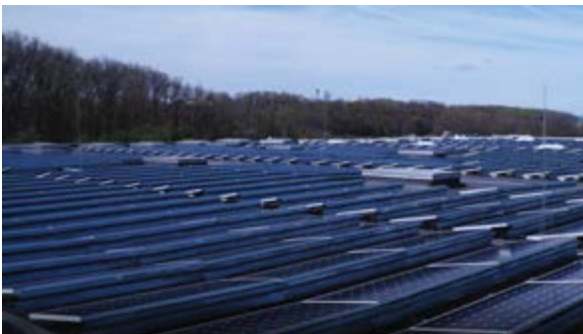
Figure 2: Phoenix Contact installed a 960-kilowatt photovoltaic (PV) array in 2021 with more than 2,600 panels at its U.S. headquarters near Harrisburg, Pa. Its monitoring system and I/O modules gather information about inverters, cameras, string currents and voltage, PV module soiling, temperature and weather, while its PLCnext controller and SCADA software aggregate, display, and transmit data to a cloud-computing service for analysis. Source: Phoenix Contact
