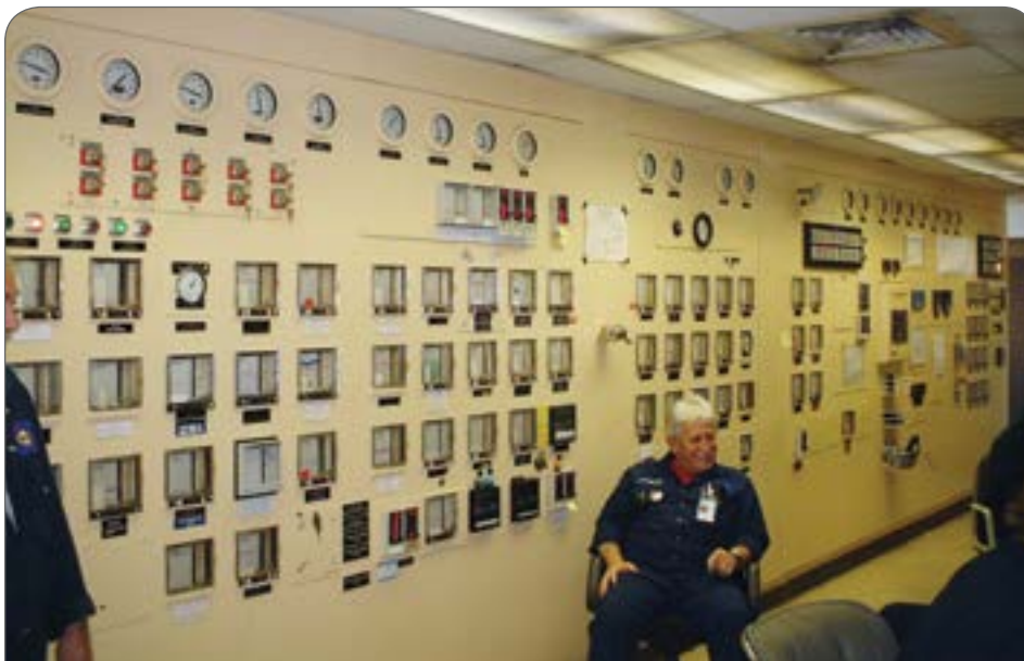
THE OLD, FAMILIAR PANEL WALL.
