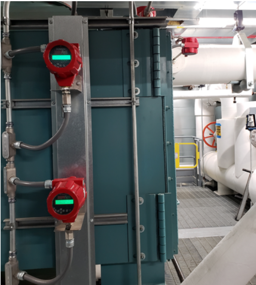
Figure 6: METER INSTALLATION Sierra Instruments' InnovaMass® 241i Insertion multivariable vortex mass flow meters measure steam – one process connection for mass flowrate, temperature, pressure, volumetric flowrate and fluid density simultaneously.
