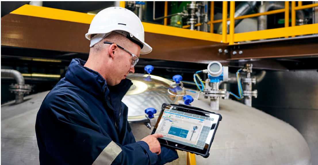
Figure 3: With Bluetooth wireless communications, a technician with a handheld device—such as an Endress+Hauser Field Xpert® SMT70 tablet PC tool can activate a proof test from up to 40 feet away from the level instrument, making it easier to perform tests on level instruments installed at the top of tanks or in inaccessible locations.
